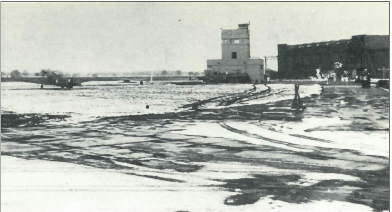
(Above) A snow covered RAF Digby during the winter of 1940 – 1941. A single Supermarine Spitfire can be seen, along with the fort style airfield control tower and a Belfast Truss type aircraft hangar.
